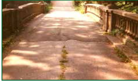
Bridge road to seminary.
